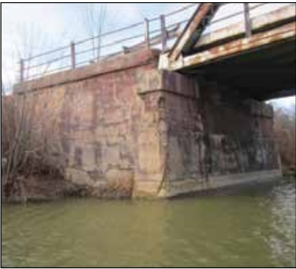
Concrete decay can be seen on the south side of the west abutment in this 2015 photo of the Holt Line Bridge.
